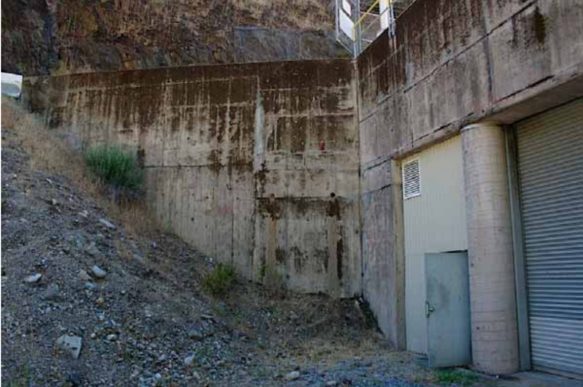
Ralston Powerhouse Garage Wall
