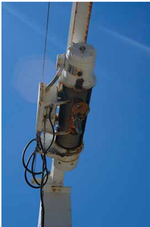
Oxbow Powerhouse - winch used as day roost
