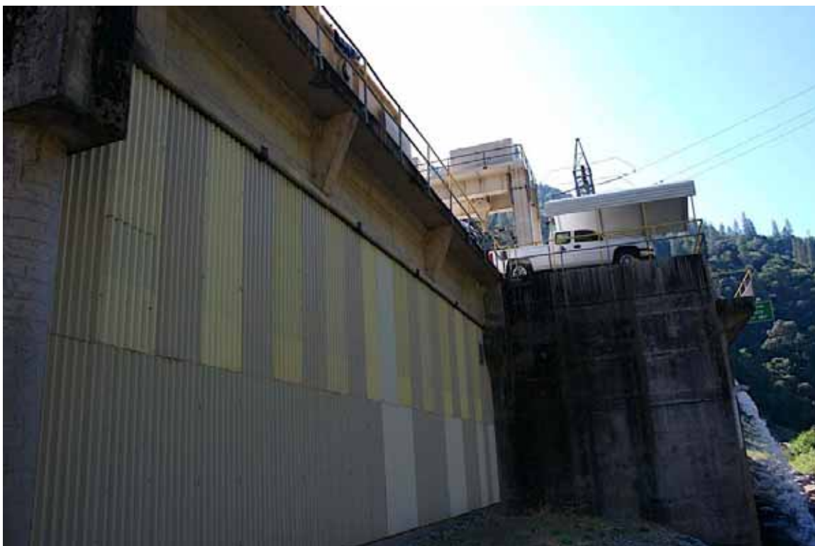
Ralston Powerhouse Garage Wall
