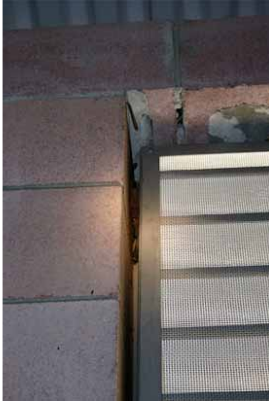
Hell Hole - Middle Fork Tunnel Gatehouse - single roosting bat inside gatehouse
