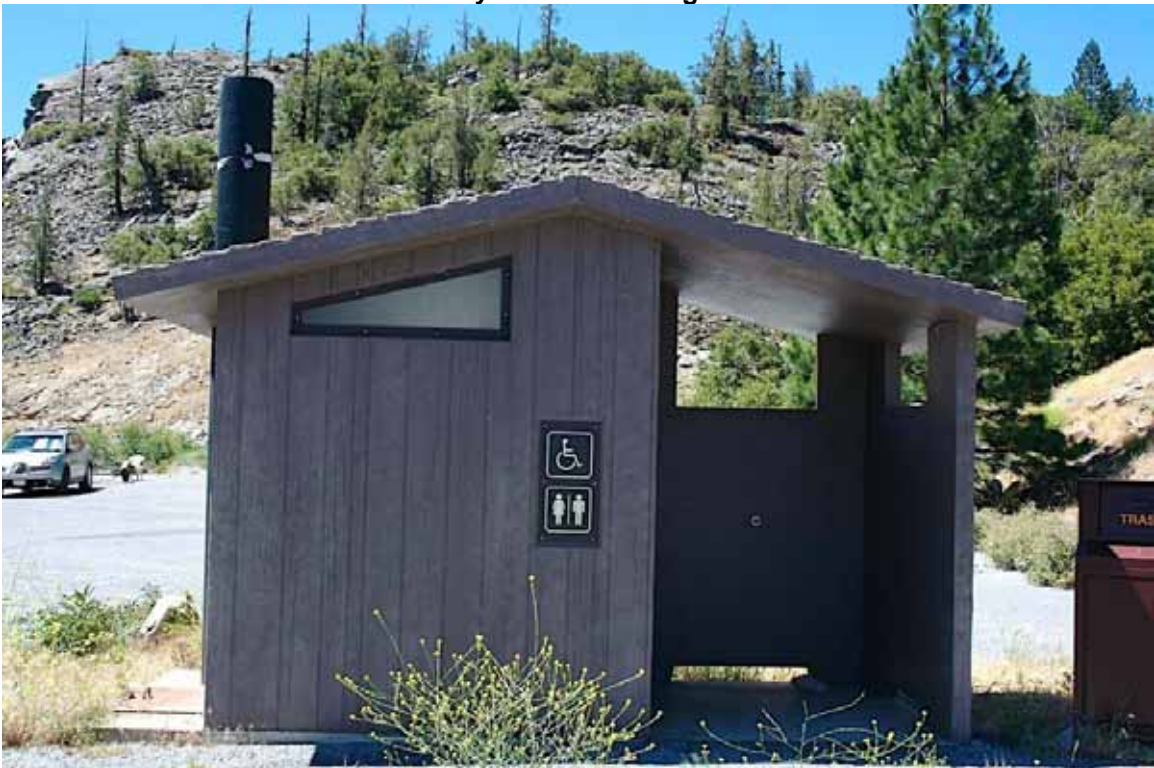
Pre-Fabricated Toilet - no suitable habitat for bat use
