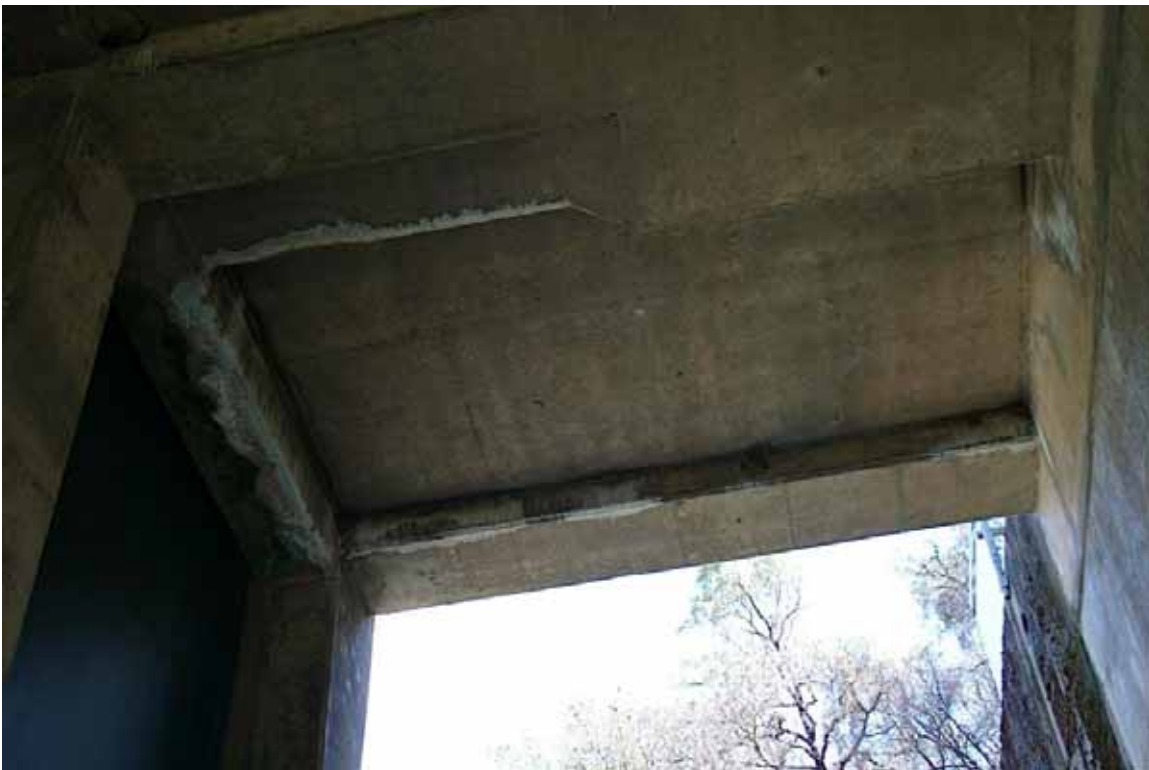
Oxbow Powerhouse - alcove ceiling
