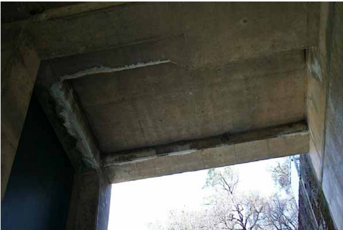
Oxbow Powerhouse - alcove ceiling
