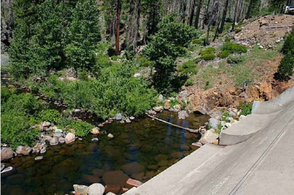
Duncan Creek Diversion Dam
