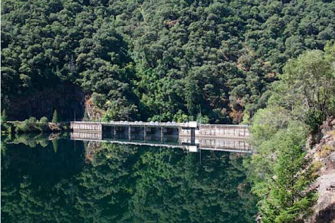
Ralston Afterbay Dam
