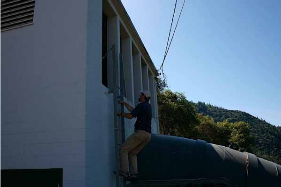
Ralston Powerhouse Penstock and Butterfly Valve House
