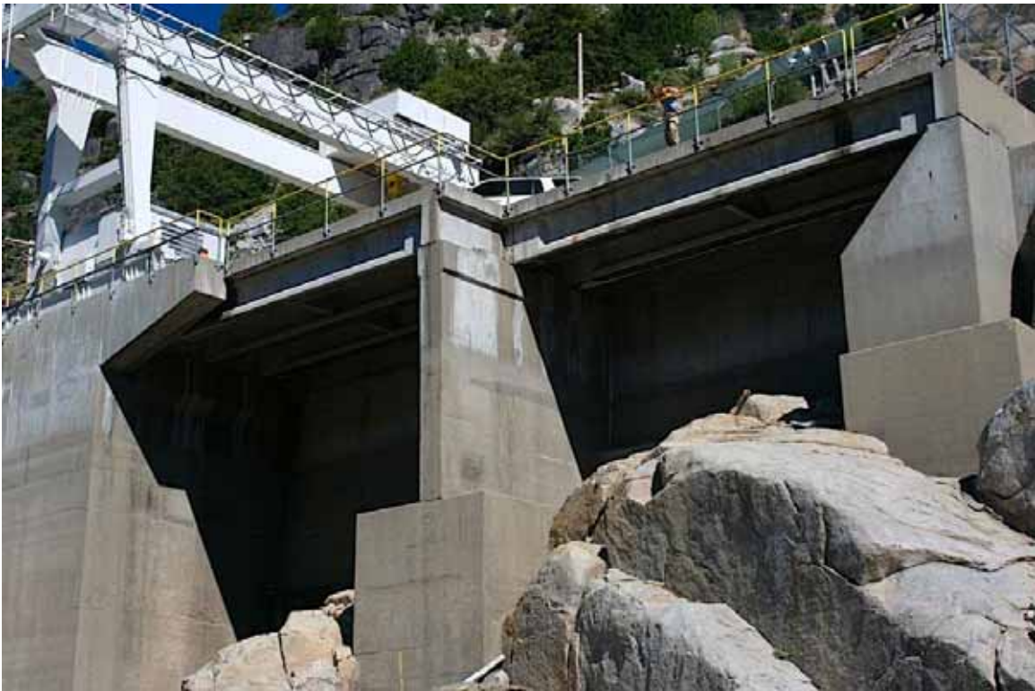
French Meadows Powerhouse - sign of extensive night roosting activity in alcoves
