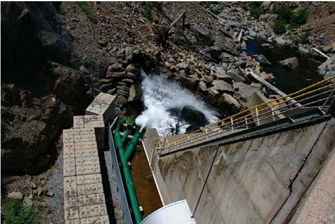
Middle Fork Interbay Dam - downstream view
