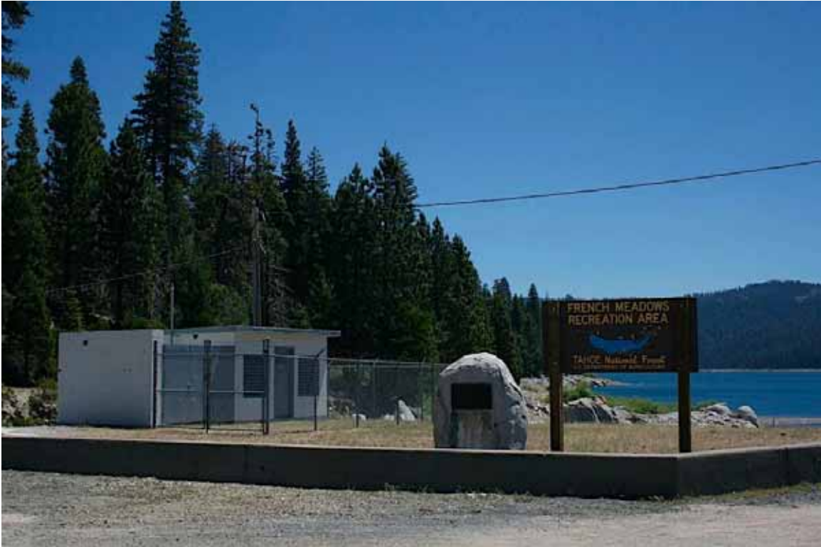
French Meadows Dam Generator Building
