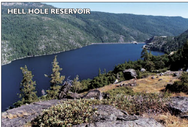
Installation of spillway gates on Hell Hole Reservoir will increase seasonal storage and power generation.
