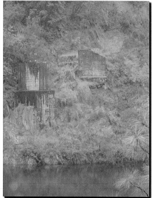
(fig. 1) Remains of the Greenwood Bridge. April 2, 2010
