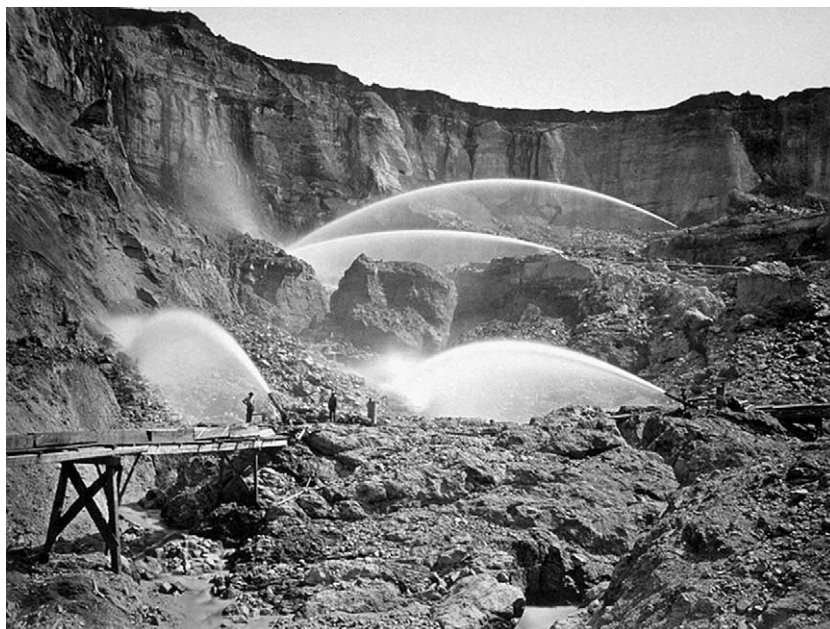
Fig. 2. Hydraulic mining at Malakoff Diggings located in the South Yuba River watershed (circa 1876). (Historic photograph taken by Carleton E. Watkins is located in the Hearst Mining Collection at the Bancroft Library, University of California at Berkeley).
