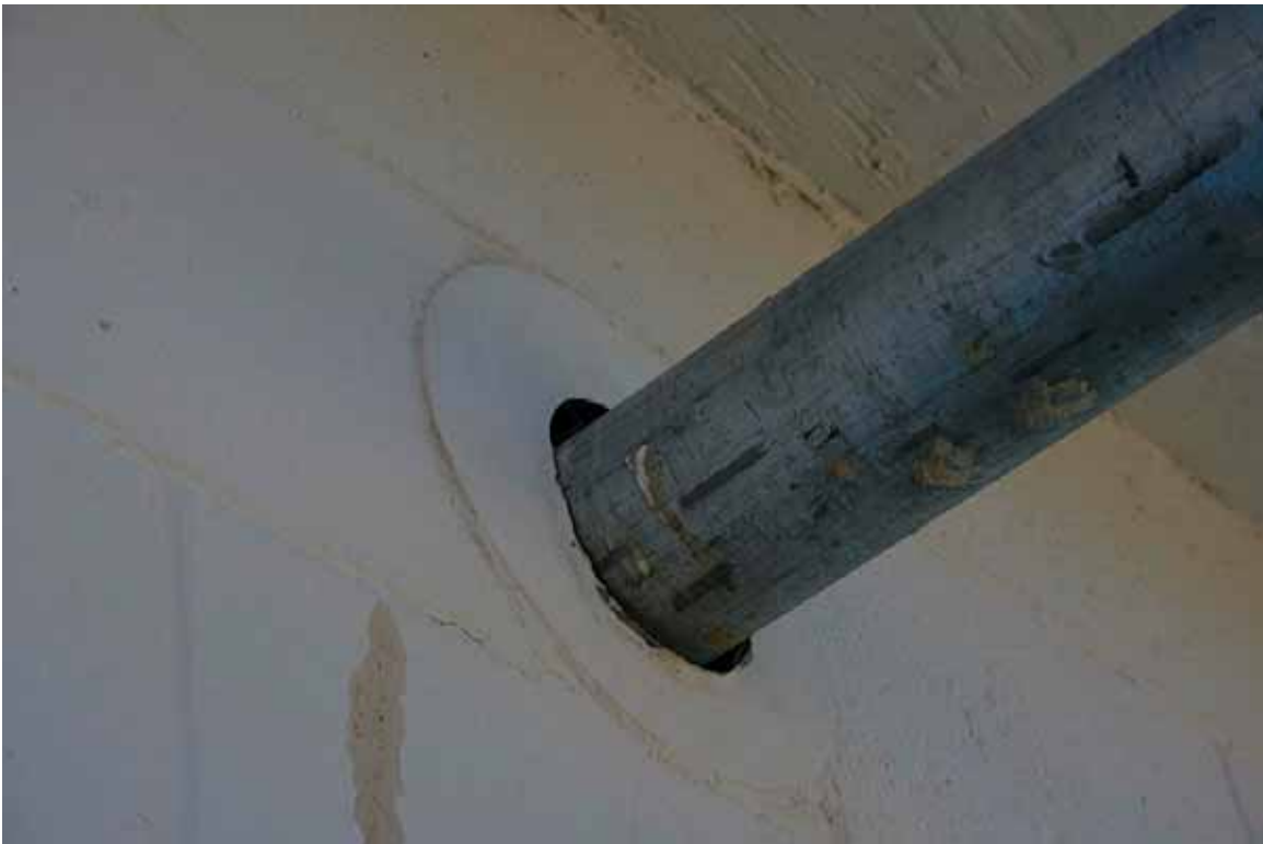
Ralston Afterbay Generator Building - bat access to interior
