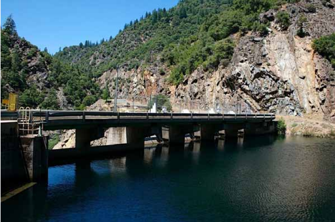
Middle Fork Interbay Dam - upstream view
