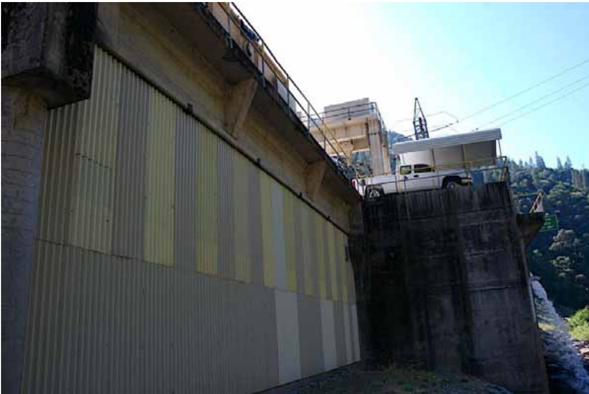
Ralston Powerhouse Garage Wall
