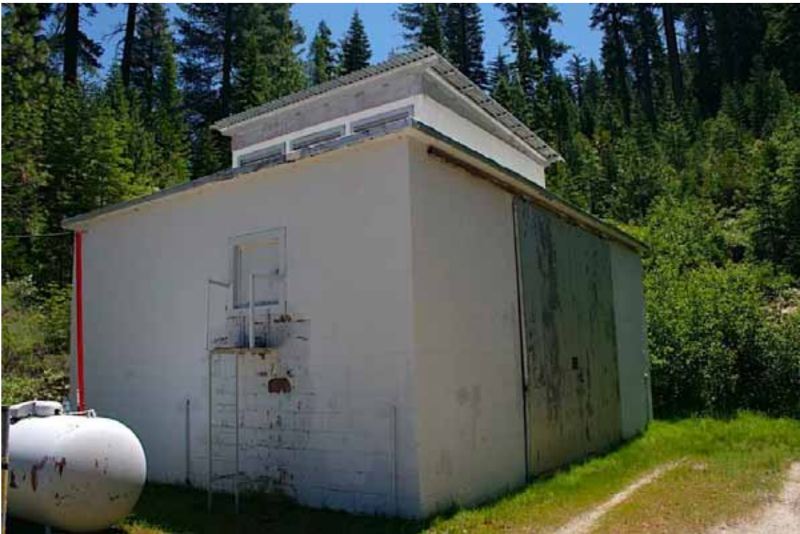
French Meadows - Hell Hole Tunnel Gatehouse
