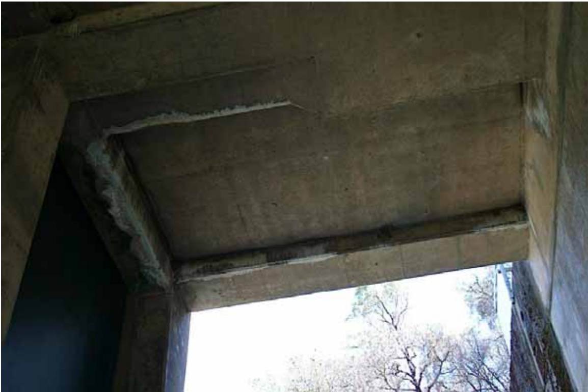
Oxbow Powerhouse - alcove ceiling
