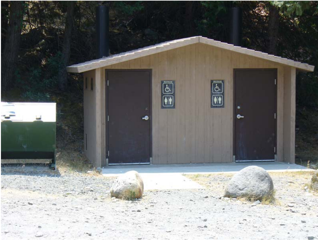
Photo T-2-7. Double unit accessible CXT and bear-proof garbage adjacent to parking area. (7/23/08)
