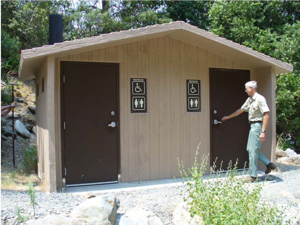
Photo T-2-8. Double unit accessible CXT upslope from parking area. (7/23/08)
