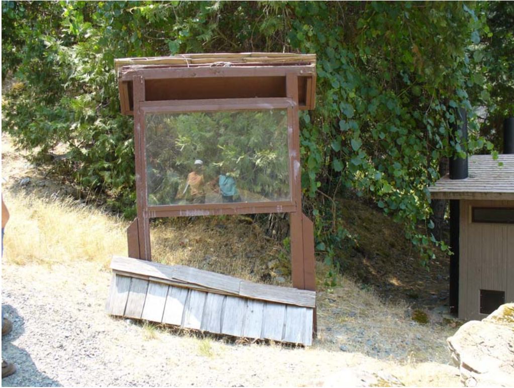
Photo T-2-9. Damaged information board adjacent to CXT upslope from parking area. (7/23/08)
