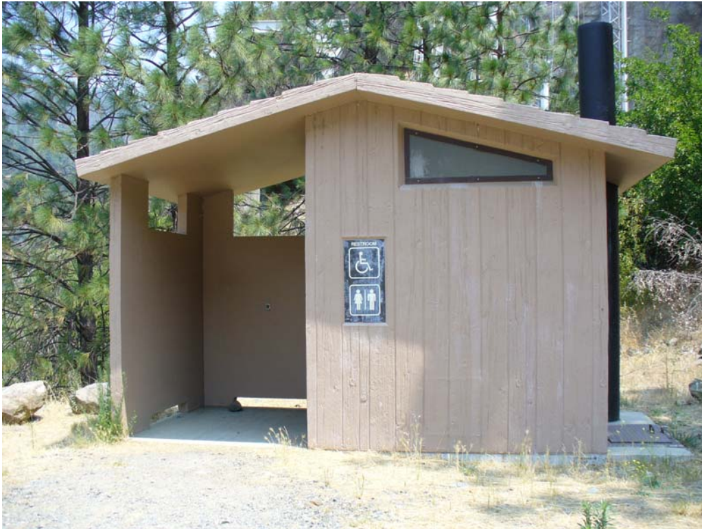
Photo T-2-6. Single unit accessible CXT adjacent to boat launch ramp.
