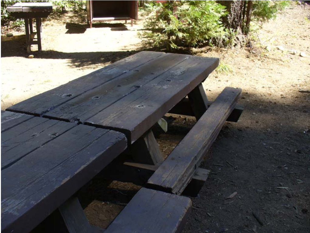
Photo R-2-12. Older picnic tables at Unit 1. All are in fair condition, with peeling paint and cracks. This one is in poor condition due to damage bench. (8/21/08)
