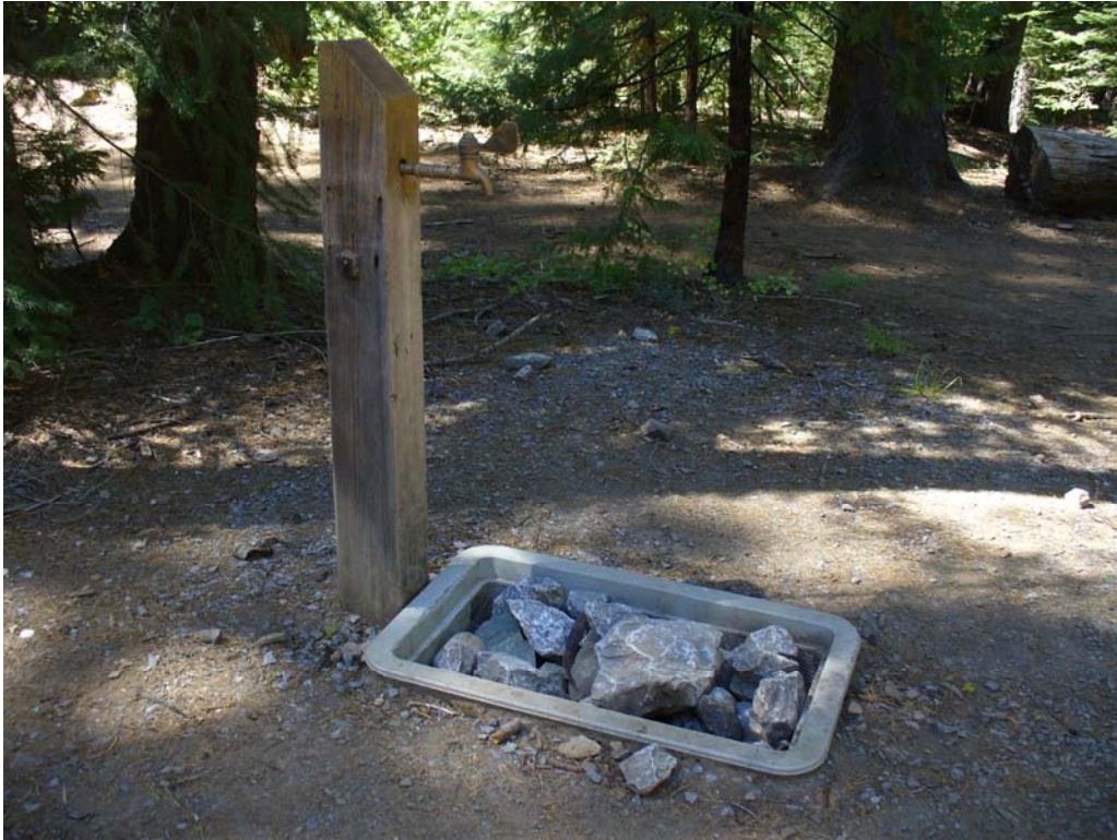
Photo R-2-19. Accessible faucet at Unit 2. (8/21/08)
