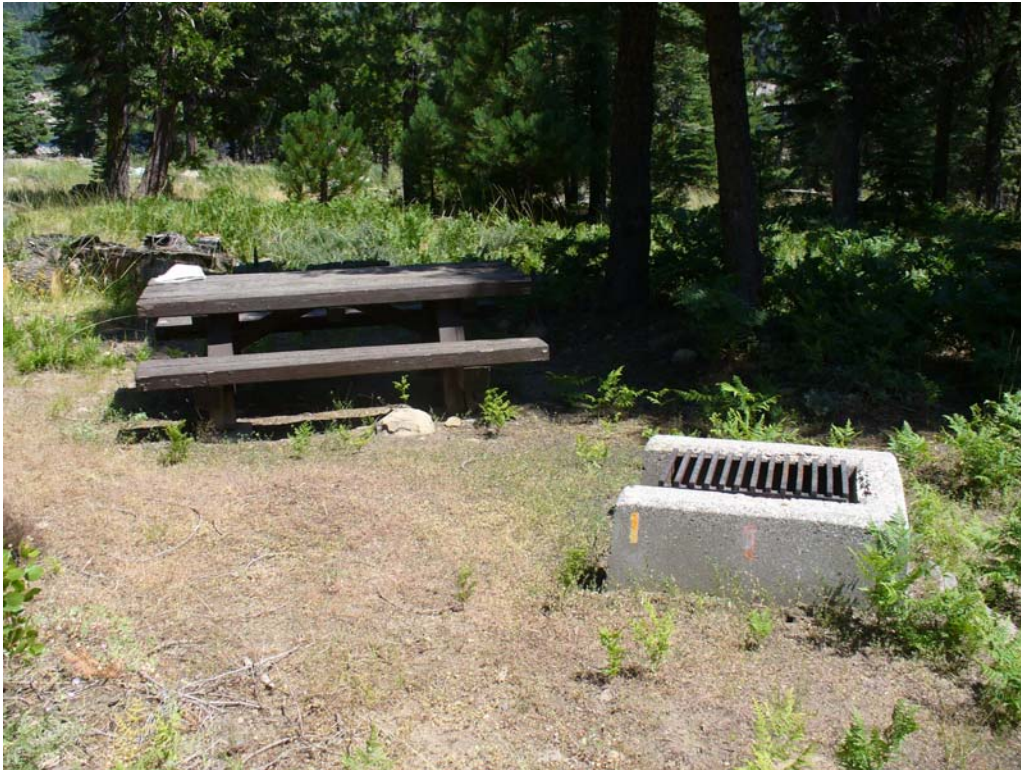
Photo Q-2-7. Typical picnic site at McGuire Picnic Area (Site 1). Note heavy wood table and concrete/steel cooking grill. Features are not disabled accessible, nor is the site due to obstacles (brush and rocks) and level changes. (7/23/08)
