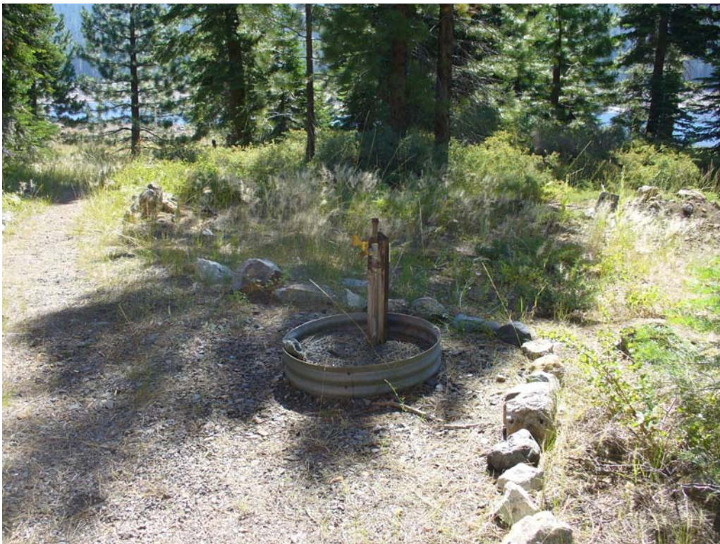
Photo Q-2-12. Water faucet located along path to McGuire Beach, near bathroom. Handle is accessible but approach is not because the sump/drain is set above grade. (7/24/08)
