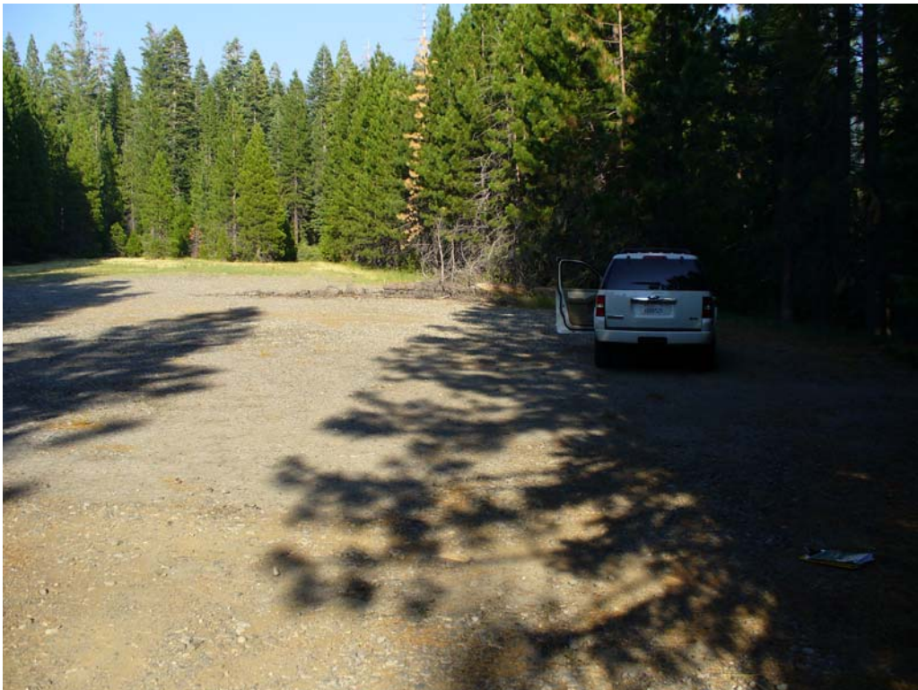
Photo P-2-6. McGuire Boat Ramp Parking Area – southeast lot. Surface has deteriorated to base rock and is in poor condition. (7/23/08)
