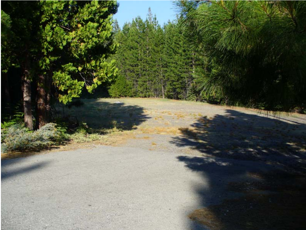
Photo P-2-8. North entrance to McGuire Boat Ramp Parking Area – northeast lot. Note transition from asphalt pavement access road to base rock in parking area. (7/23/08)
