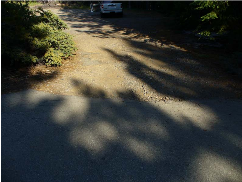
Photo P-2-5. Entrance to McGuire Boat Ramp Parking Area – southeast lot. Note transition from asphalt pavement access road to base rock in parking area. (7/23/08)
