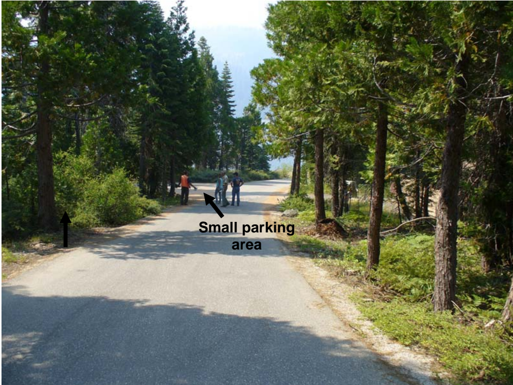
Photo O-2-8. Paved road extending from French Meadows Boat Ramp Parking Area to French Meadows Boat Ramp. Note small parking area on left side of road. This area also functions as a high water turn-around at max WSE. (7/23/08)
