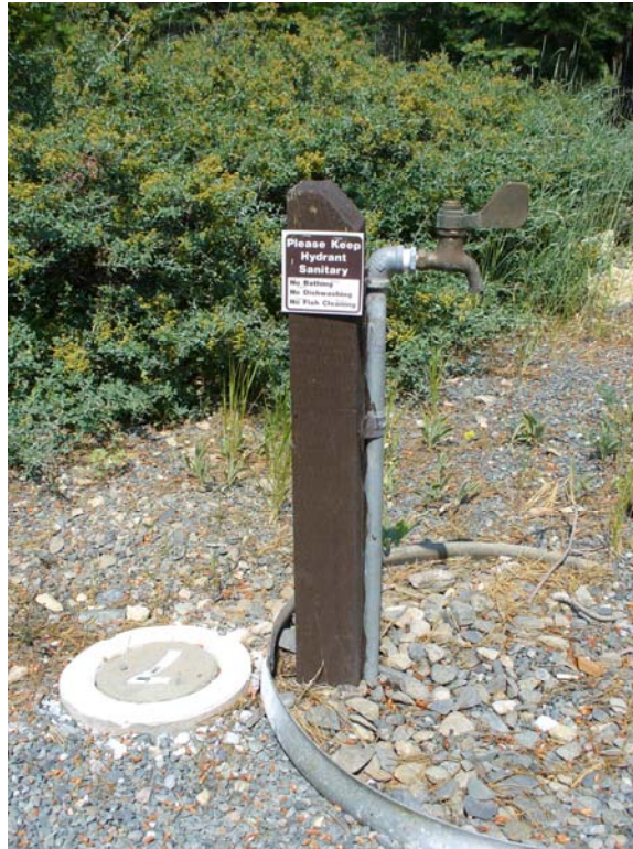
Photo O-2-11. Water faucet located adjacent to bathroom. Handle is considered disabled accessible. Approach is not disabled accessible due to insufficient clear space and changes in surface level. (7/23/08)
