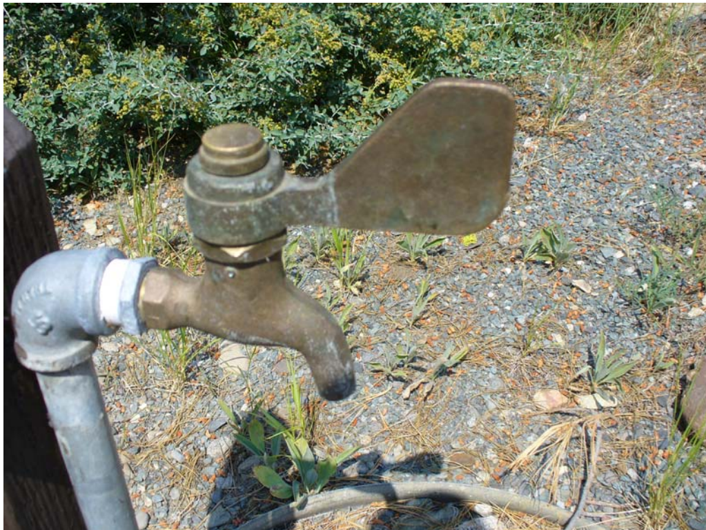
Photo O-2-12. Example of disabled accessible faucet handle.
