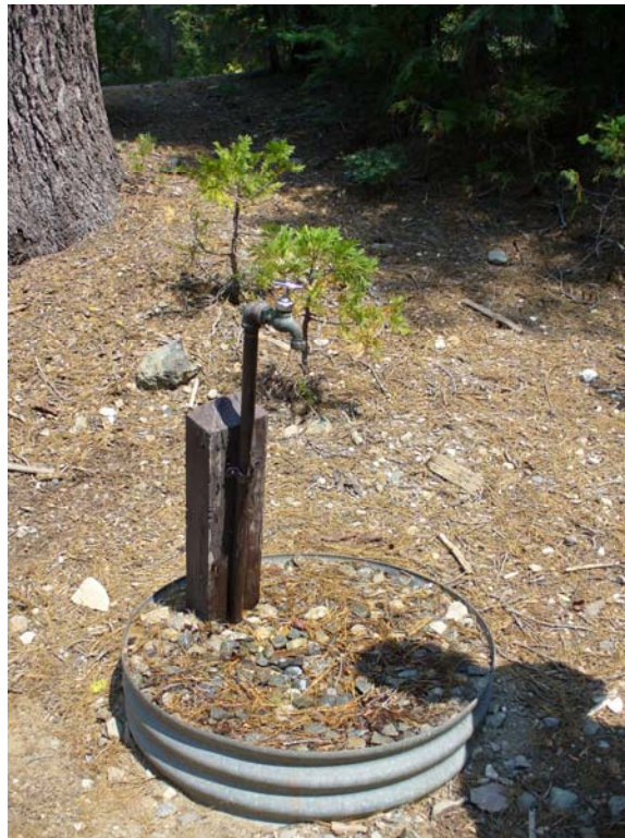
Photo O-2-18. Water faucet near vault toilet. Does not meet accessibility standards due to handle design, obstacles, and level changes. (7/23/08)
