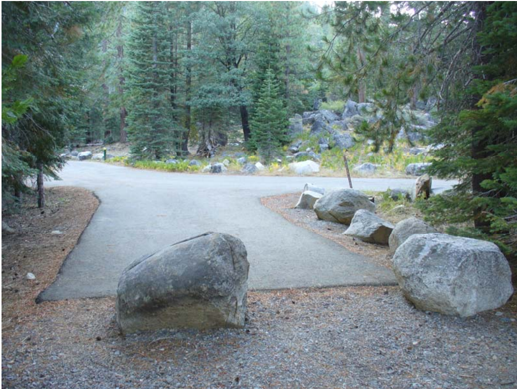
Photo N-2-15. Turn-around area at Lodgepole. Note pavement is in good condition. (9/408)
