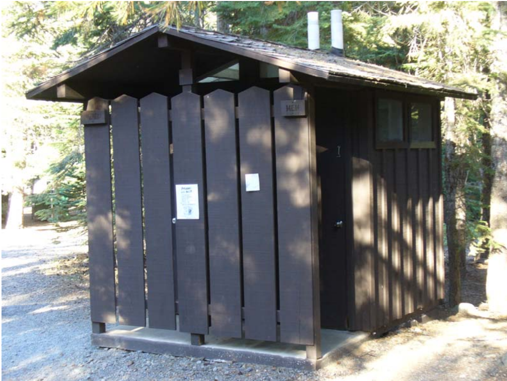
Photo N-2-9. Typical vault bathroom in Gates Group Campground. This bathroom is located in Ponderosa Campground. None of the bathrooms in the Gates Group Campground are accessible. (9/4/08)
