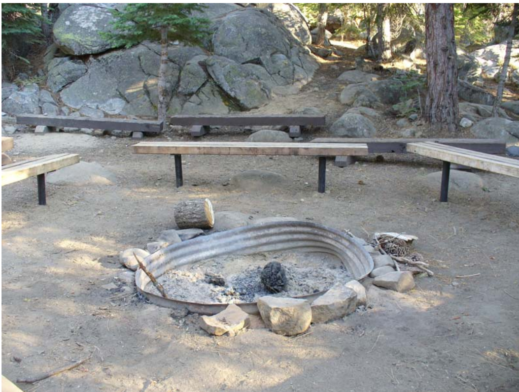
Photo N-2-14. Damaged group fire pit at Ponderosa. Note new benches in middle ground and old benches in background. (9/4/08)
