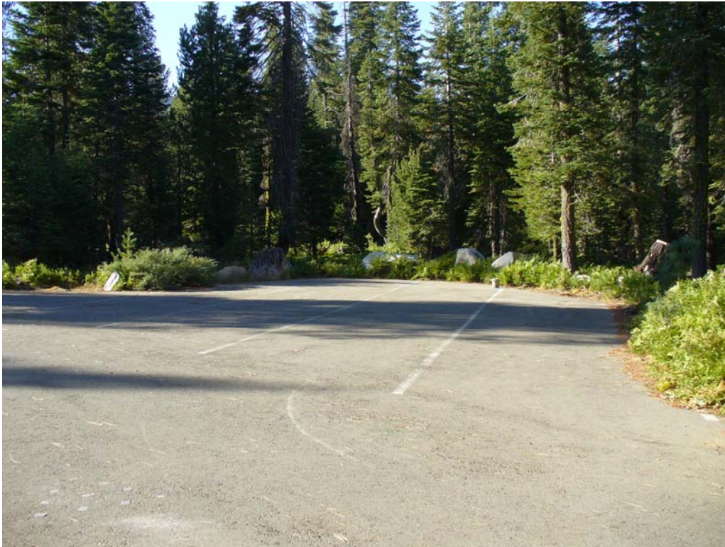
Photo N-2-7. Typical parking area at Gates Group Campground. This parking area is located at the entrance to Ponderosa. Note the striping and long stalls for trailers/RVs. Pavement is in good condition. (9/4/08)
