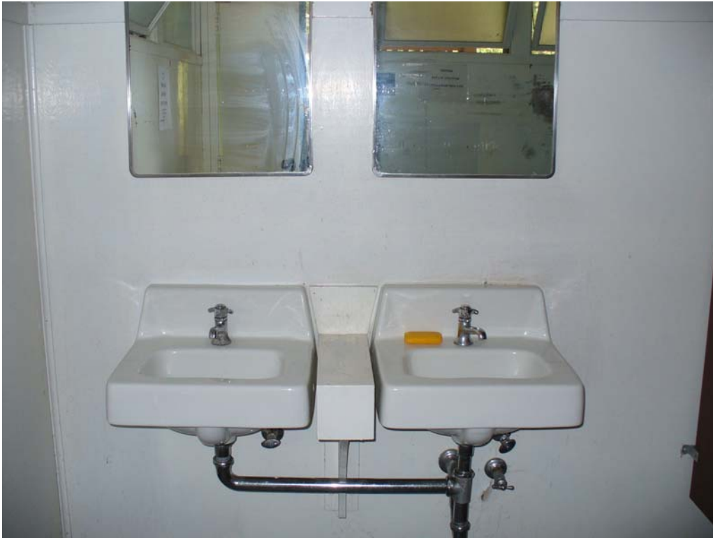
Photo K-2-13. Sinks inside of wood bathroom. (9/04/08)
