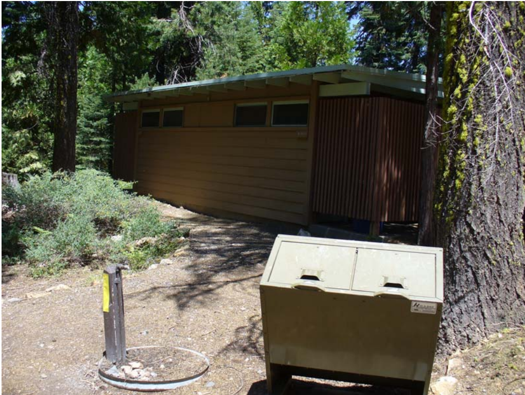
Photo J-2-17. Typical bear-proof garbage container and water faucet. Bathroom #6 in background. (7/24/08)
