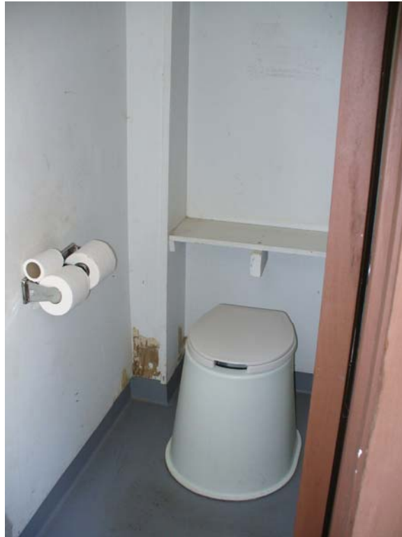
Photo J-2-15. Inside of bathroom #3. (7/24/08)
