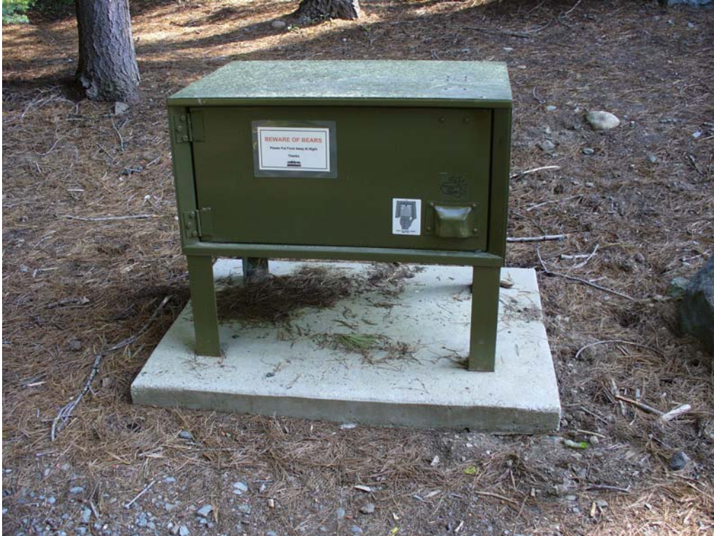
Photo J-2-18. Typical bear-proof food storage locker (bear box) on concrete pad. (7/24/08)
