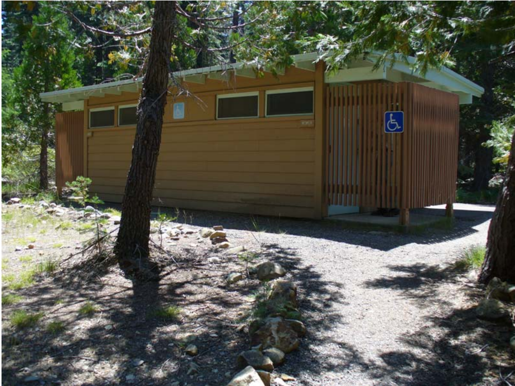
Photo J-2-10. Wood bathrooms with have flush toilets and sinks, converted to be accessible. Note accessible pathway. (7/24/08)
