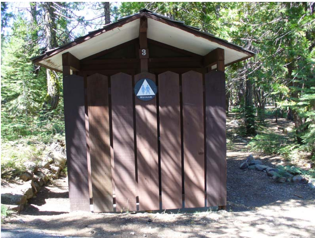
Photo J-2-14. Example double unit wood bathroom #3, not accessible. (7/24/08)
