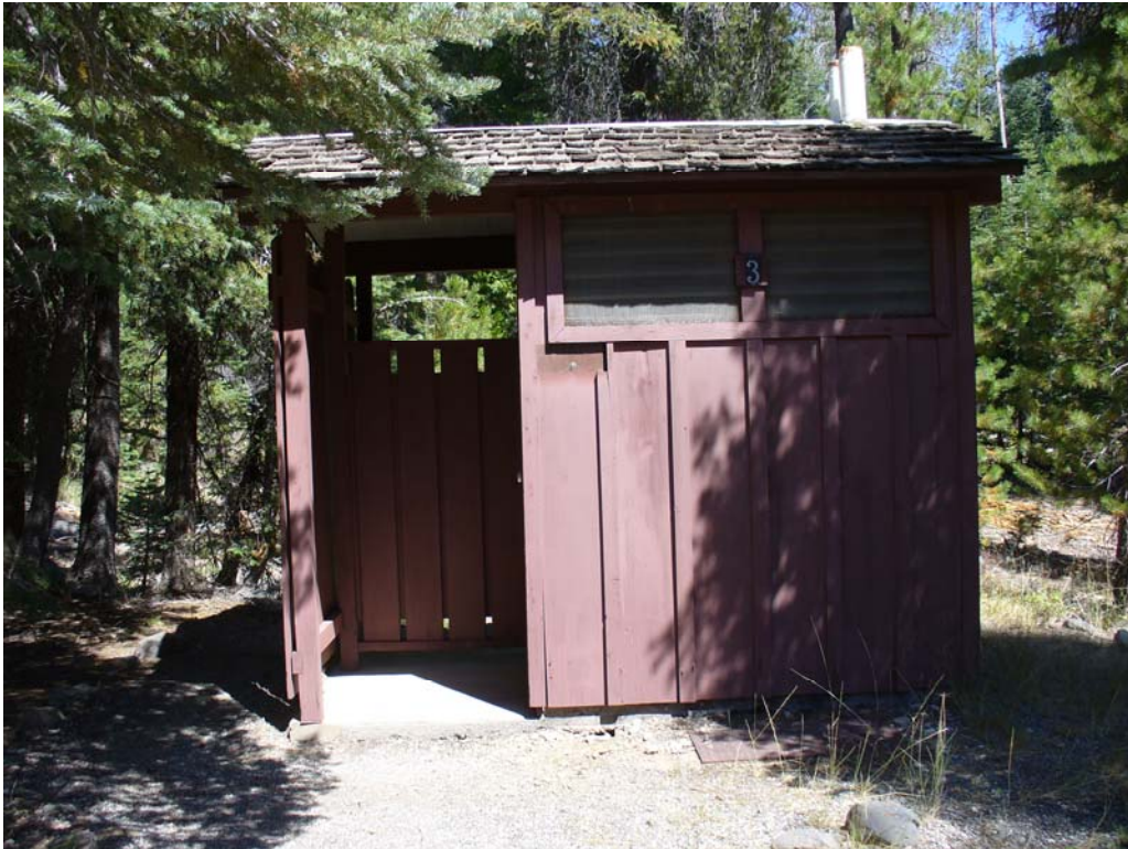
Photo I-2-15. Toilet building No. 3. (9/04/09)
