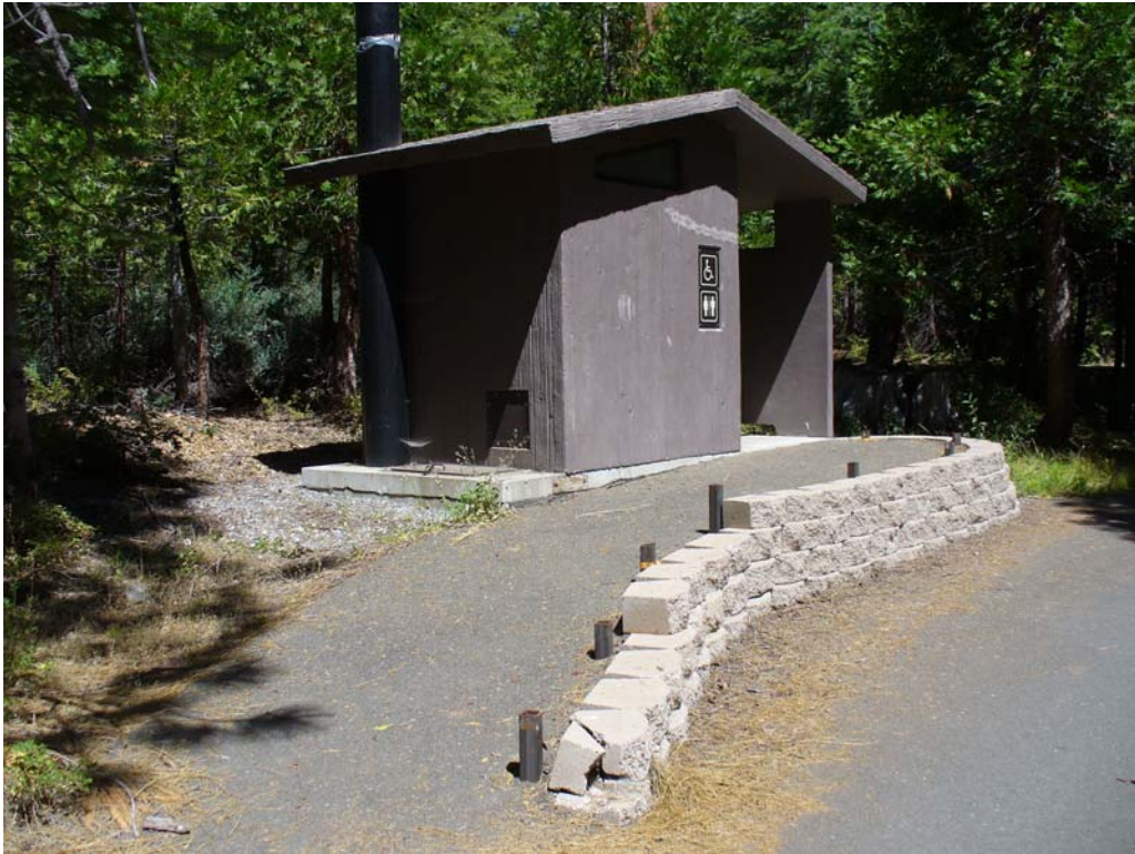
Photo D-2-15. New single-unit, pre-cast concrete toilet (CXT) – accessible. Note that ramp is missing handrail. The handrail was added later in 2008.
