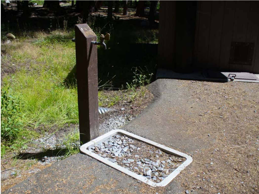
Photo D-2-16. Example water faucet - accessible (8/21/08)
