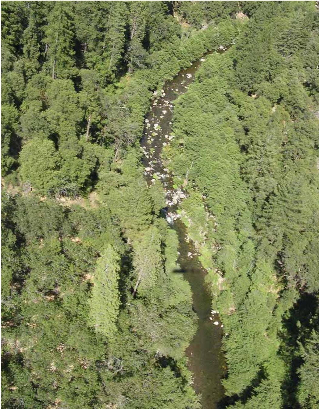
Photo E-3: Coarse Material in Channel at Base of Active Rockfall in Middle Fork American River – (RM 30.2)
